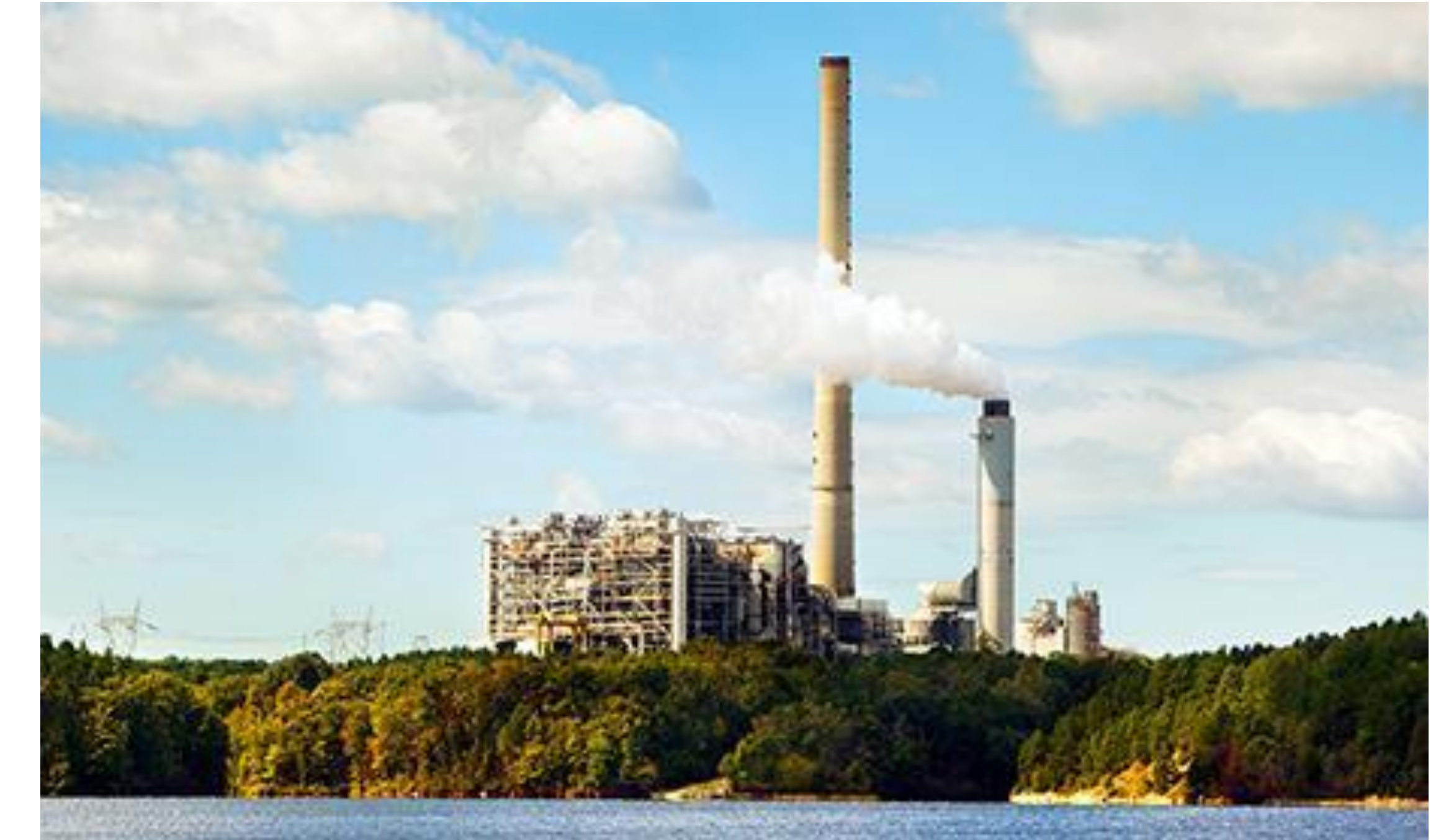
Duke Energy Mayo Steam Station
